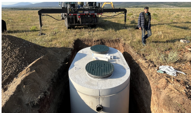
Septic System Installation
