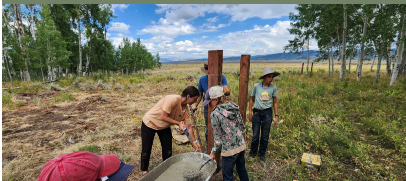
Fencing Installation Near Welcome House
